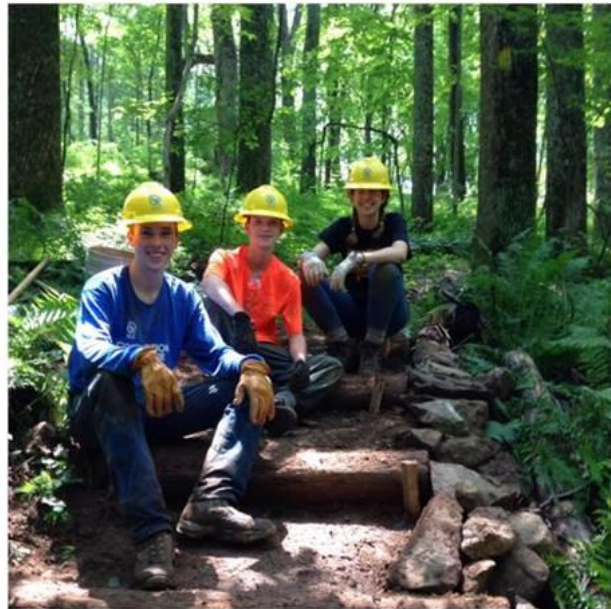
The crew enjoying their finished timber stairs project.
